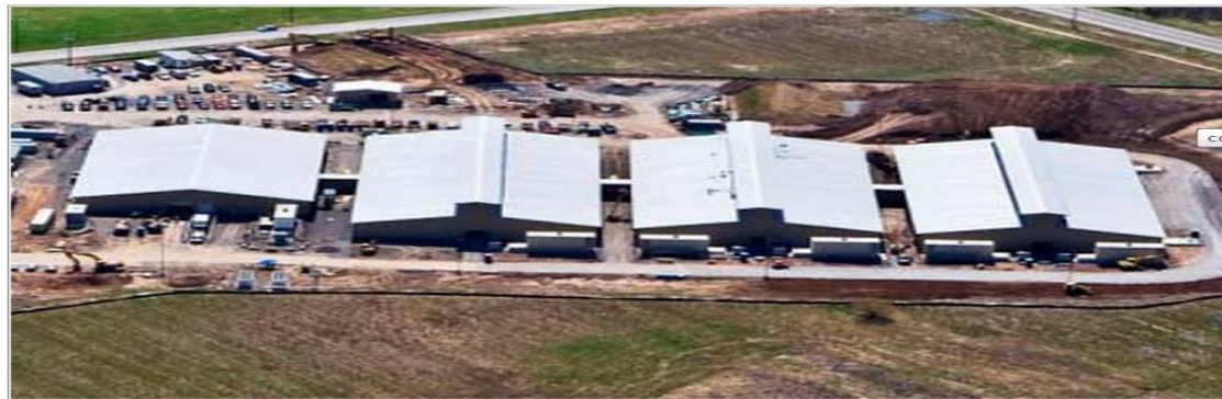
An aerial view of the Yahoo Computing Coop data center in Lockport, N.Y. Yahoo has announced plans to invest $500 million in additional data centers.
